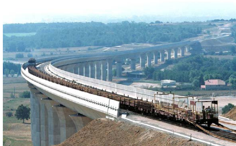
Train de chantier (source RFF)
