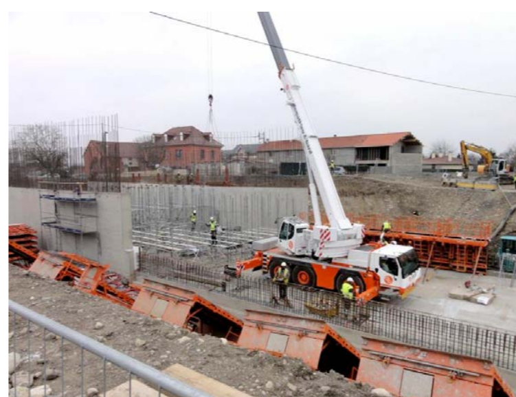
Grue mobile (Source : RFF)
